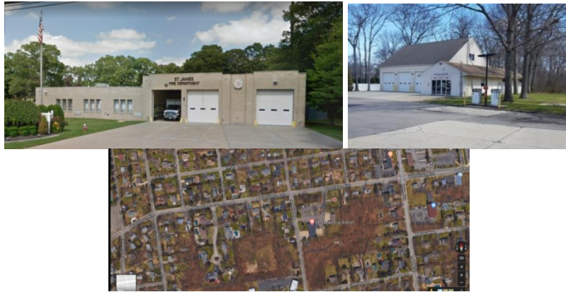
Figure 10 St James Fire District Station 2 - “3” 221 Jefferson Ave
